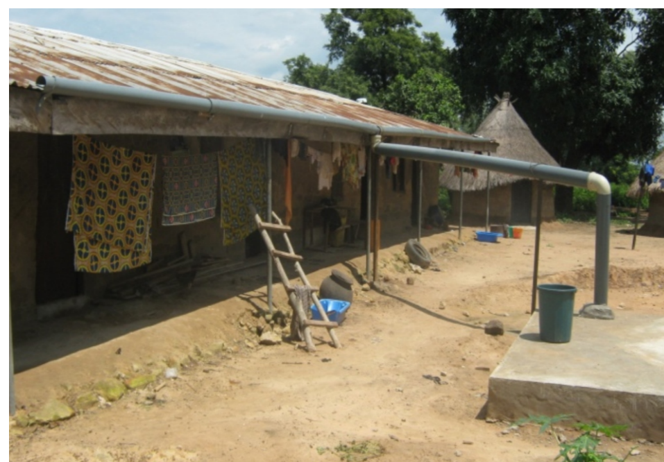
Rainwater harvesting to underground tank in Daudu
