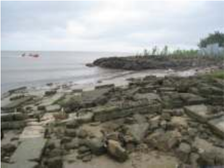
Rising sea level destroyed houses in Ibuot Utan, Mbo LGA, Akwa Ibom State
