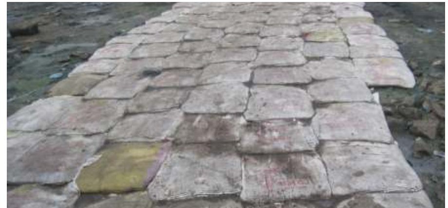
Filled sand bags to control erosion and sea level rise in Mbaka community
